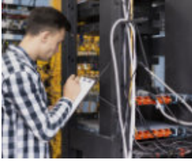
IT Panels, Server rack cabinets
